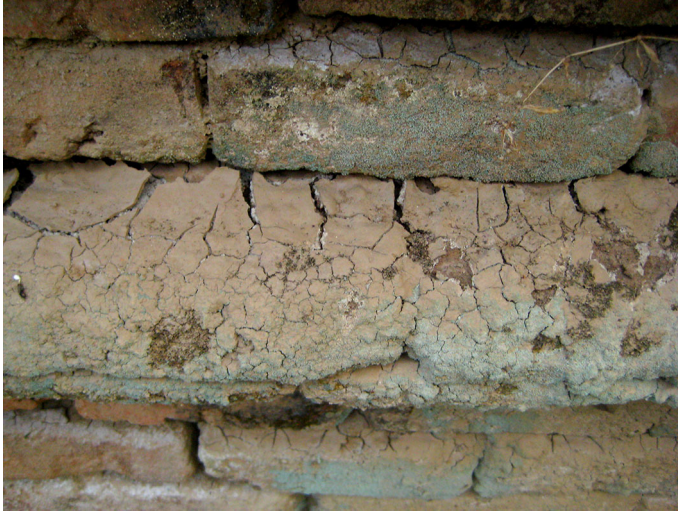
Fig. 7 Clayey-silt deposits of the 2011 Ping River flood at Wat Meng Rai in the study site
