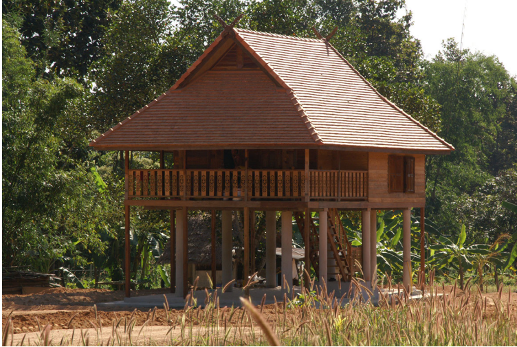
Fig. 2 An example of a traditional northern Thai house. A ‘soft layer’ is created at the bottom as the house is propped up on stilts, partly for flood mitigation. Rooms are located, and belongings are stored in the second level
