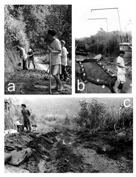
Figure 2. (a) Karen villagers repairing ruts on the road to Pang Khum by removing material from the cutslope; (b) Lisu man, Asuh, standing in front of the FILL plots and rainfall simulator; (c) Lisu man, Asam, standing beside a section of the Lower PKEW Road following the TRUCK simulations
