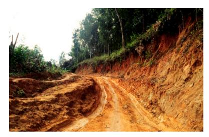
Figure 3. Surface lowering on the main road to Pang Khum. The >0.5 m elevated bench on the left was the original road surface before the rainy season began four to six months earlier
